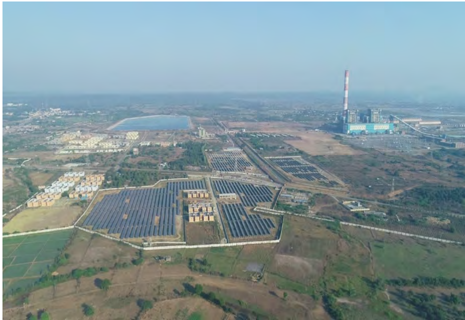
Solar Power Plant at STPP (10 MW)
