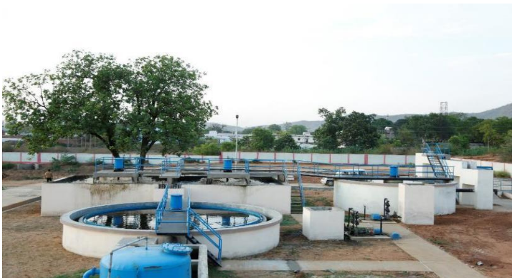
Figure 5.4: 0.8 MLD STP at Block-B, NCL
