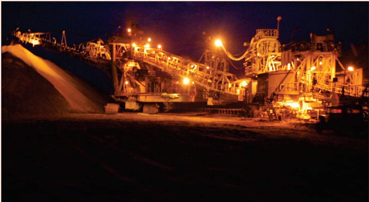
Spreader at OCP-II Project, RG-III Area
