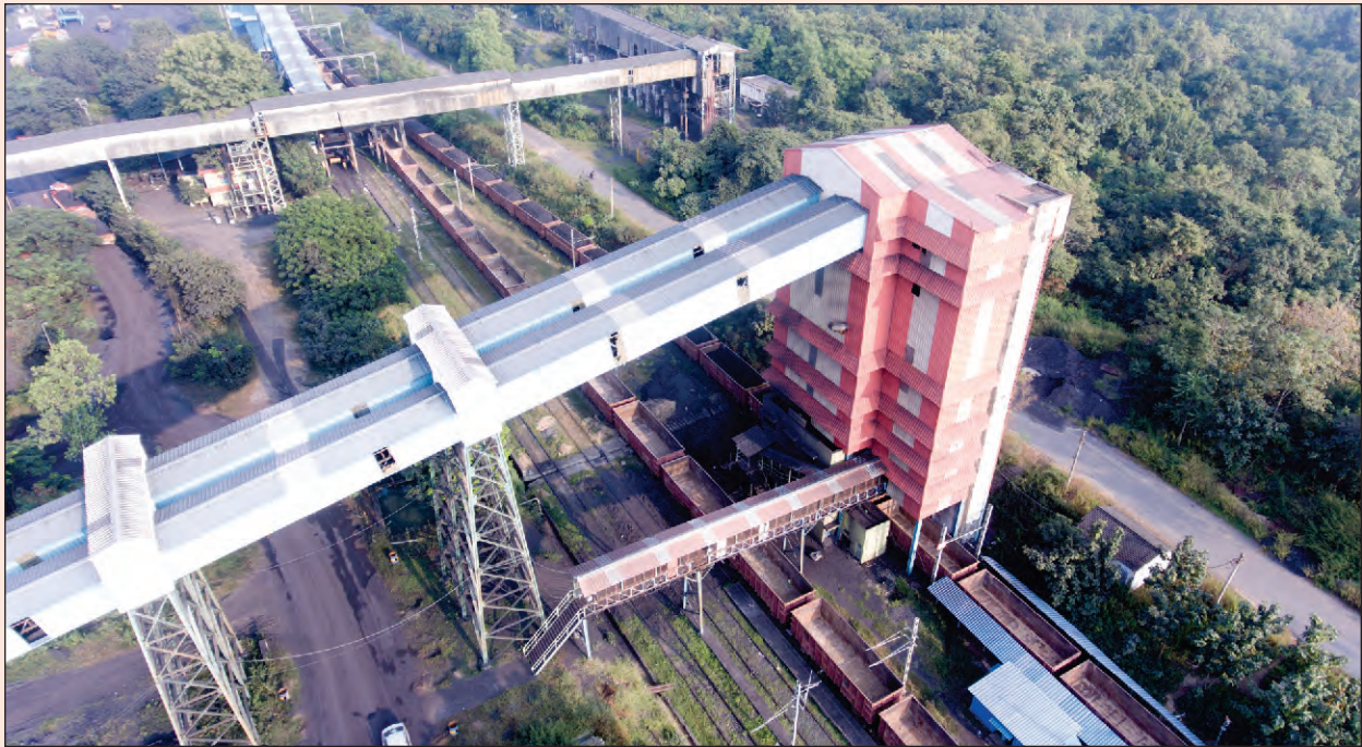
Coal handling plant
