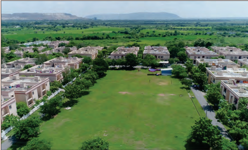
Integrated SCCL Township for employees
