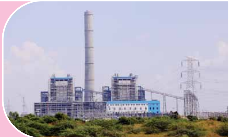
Singareni Thermal Power Project, Jaipur Mandal, Adilabad Dist.,
