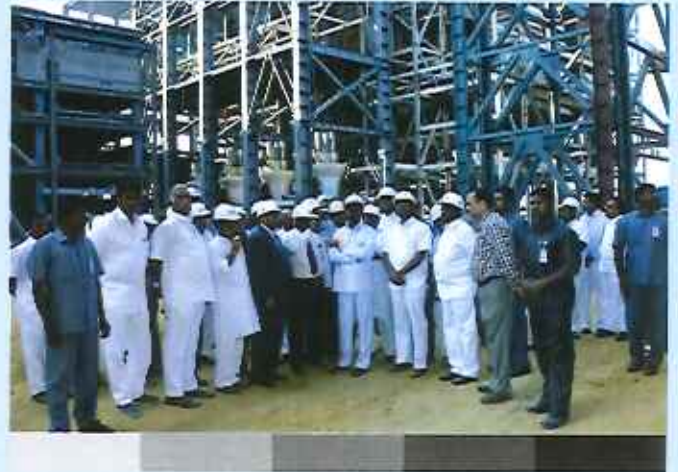
Hon'ble Chief Minister reviewing progress of 2x600 MW Thermal Power Plant under construction at Jaipur (V) in Adilabad district
