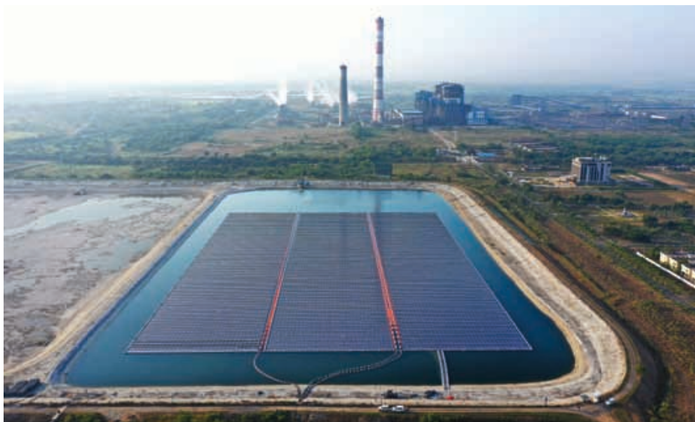
5 MW Floating Solar Power Plant at STPP
