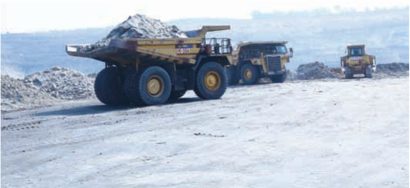
Back filling activity in Open Cost Mines (RG OC-1, RG 3 Area)
