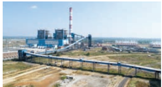
Singareni thermal power plant (Jaipur) Mancherial
