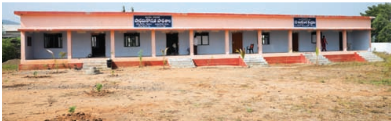
Primary School Building Constructed at New Padmagudem Village with Singareni CSR Fund
