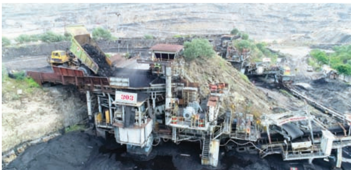
Input Crusher and Conveyor Technology in OC-1 Mine of RG-3 Area
