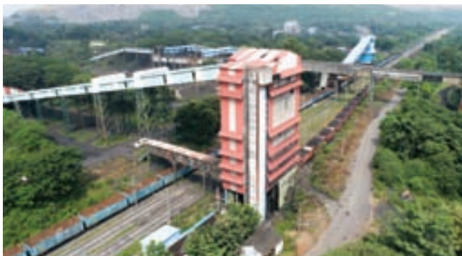
KCHP at Manuguru area
