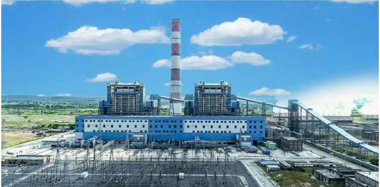
PANORAMIC VIEW OF POWER PLANT
