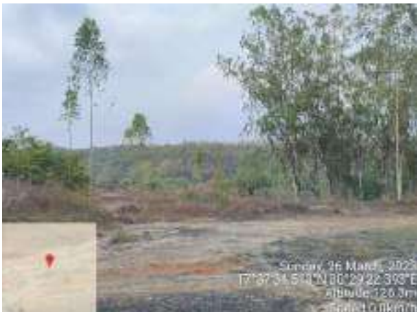
Backfilling area Under reclamation
