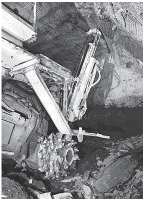
Fig. 11 Sandvik bolting rig on roadheader MR620
