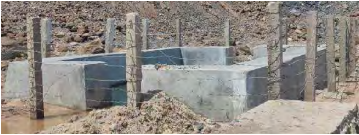
Figure 6.5: Catch drain & Siltation pond at Top Soil & OB dump, Amrapali OC, CCL
