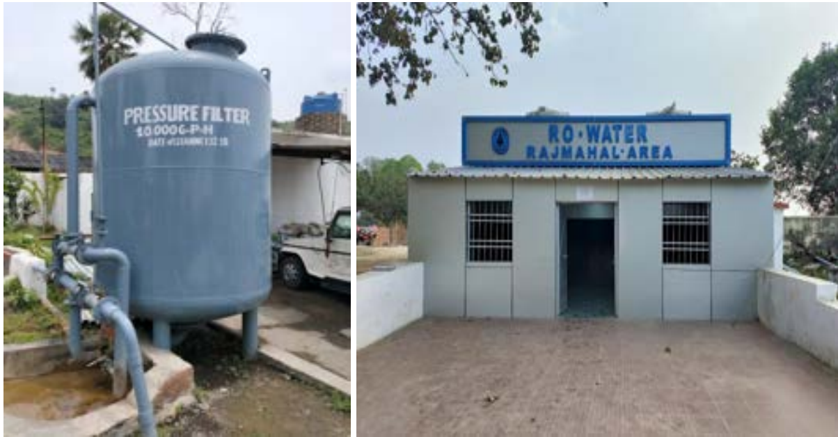
Figure 7.6: Pressure Filter and RO Water Facility at Rajmahal Area, ECL
