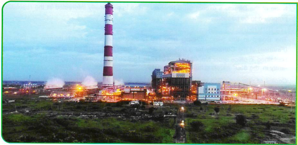
Night View of The Singareni Thermal Power Project (2x600 MW), Jaipur, Mancherial Dist.
