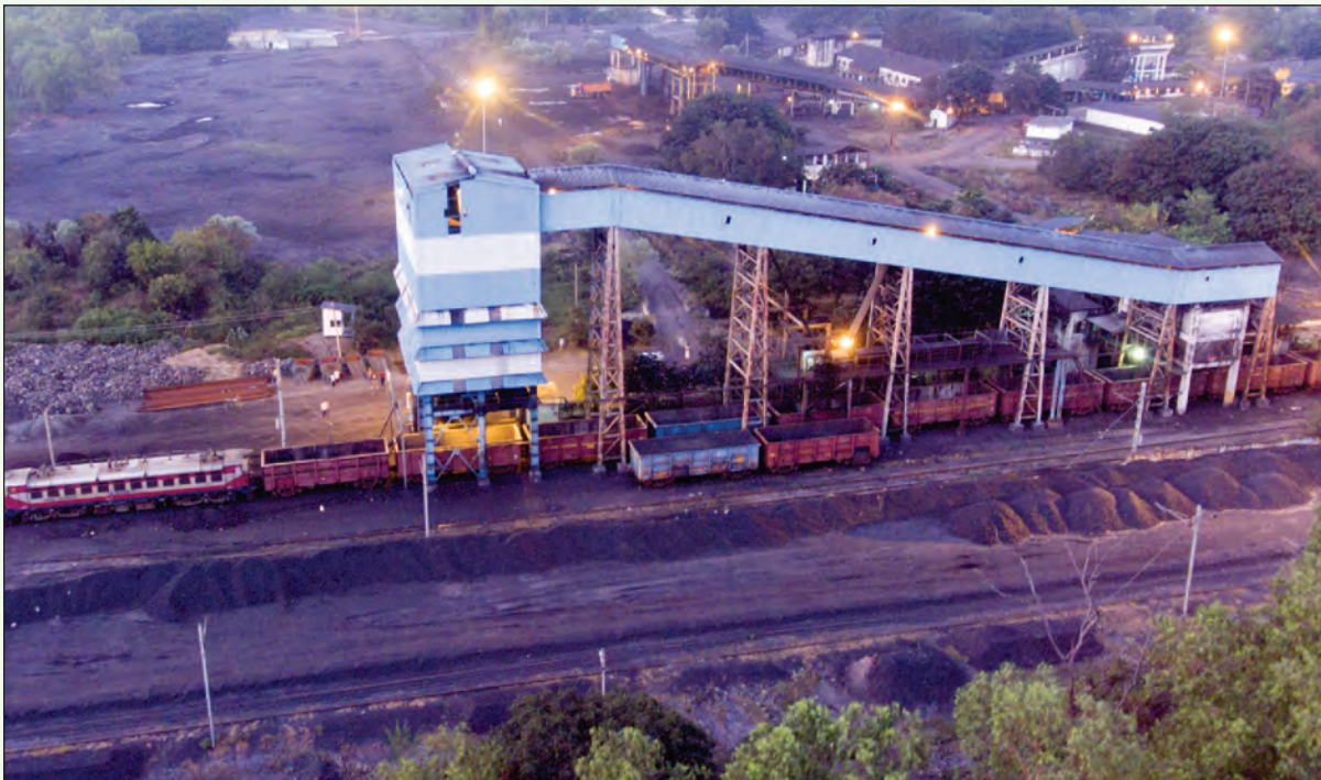
Coal handling plant at Srirampur – Biggest in Singareni
