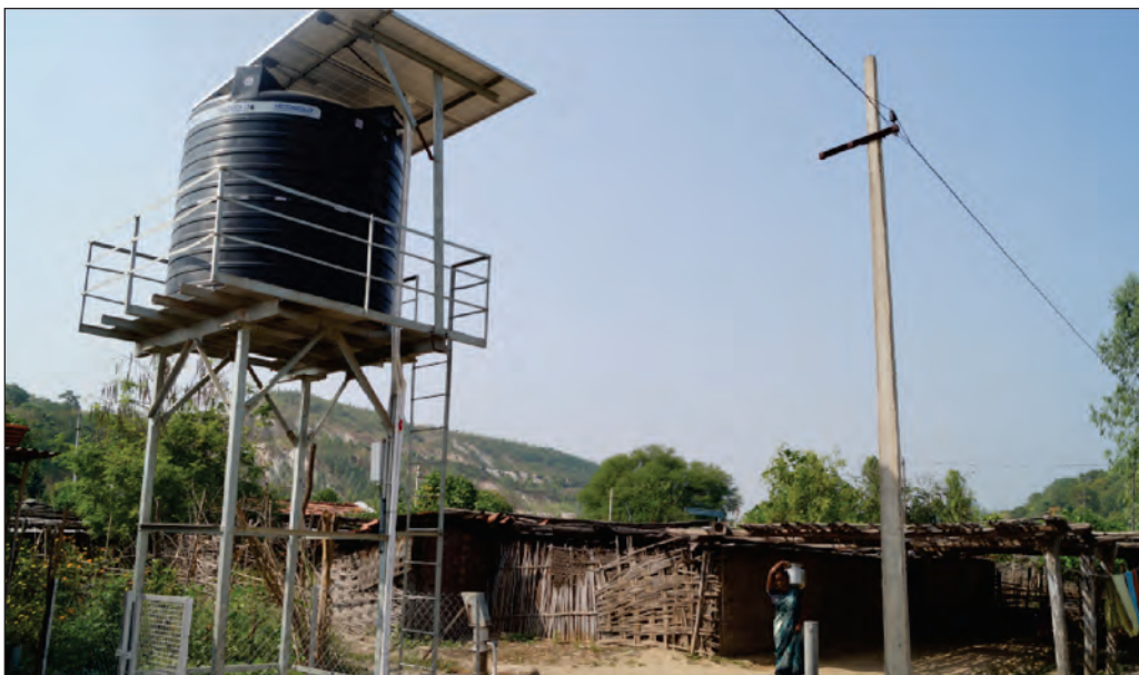
Solar powered drinking water facility provided at Ontimamidi R&R centre, Belampalli
