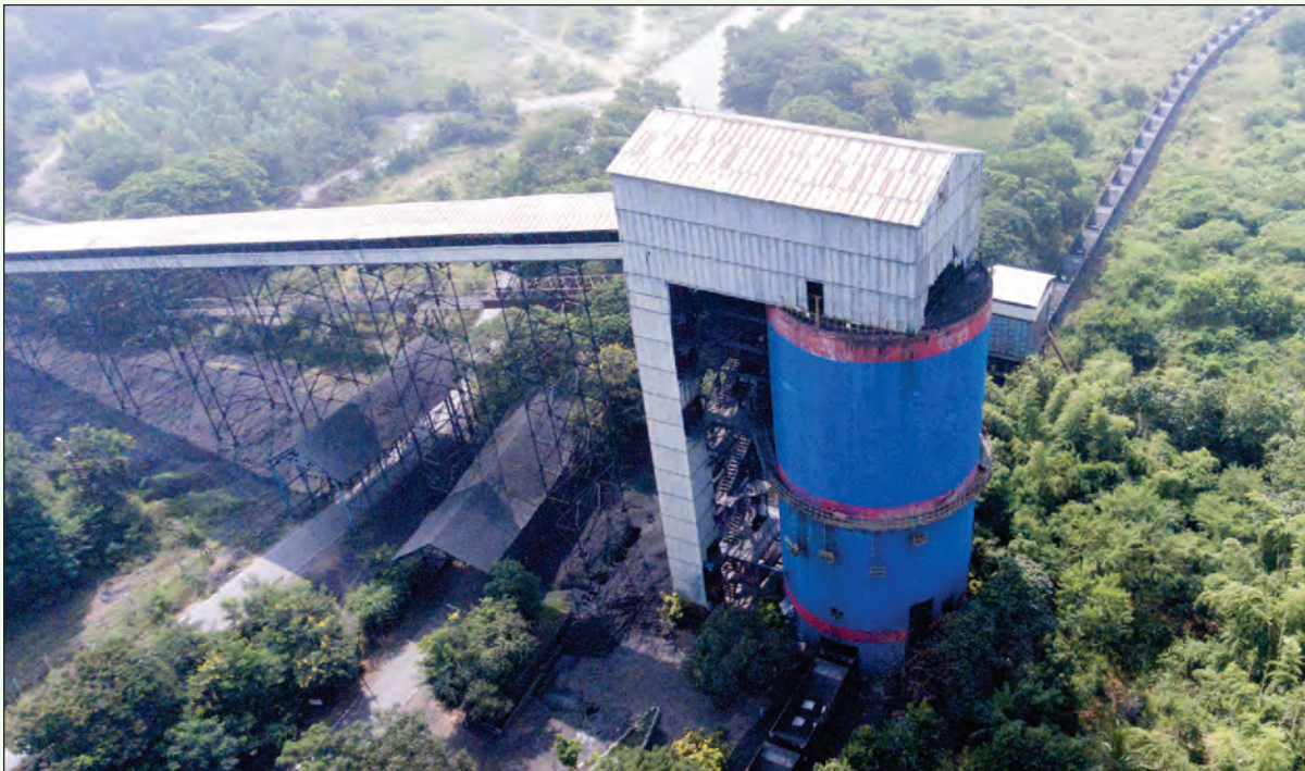
Silo at RG-II area for dispatch of coal to NTPC
