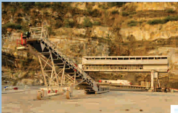
Pioneering Technology - working of Highwall Mining at Ramagundam OC-II Project
