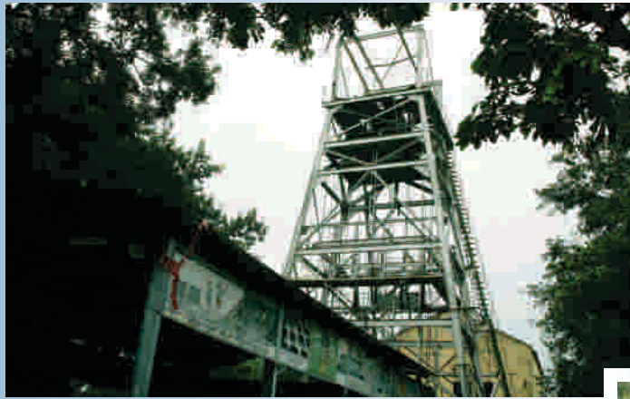
Manwinding arrangement at Venkatesh Khani, Kothagudem
