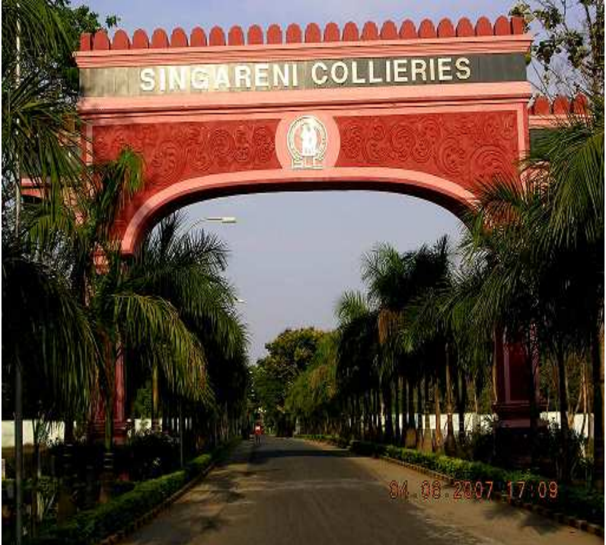
A WELCOME ARCH AT BUNGALOWS AREA, KOTHAGUDEM
